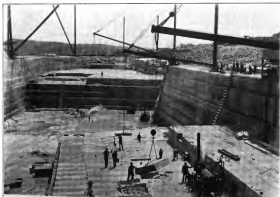
HANDLING HEAVY BLOCKS IN THE BEALER QUARRY
